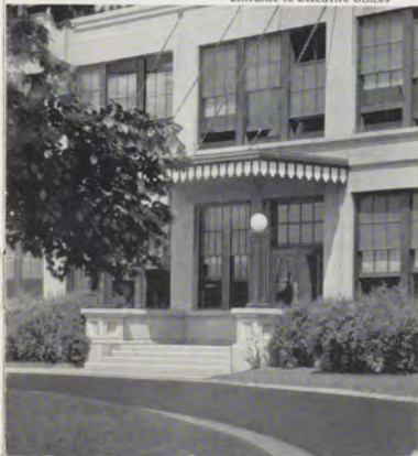
Entrance to Executive Offices
