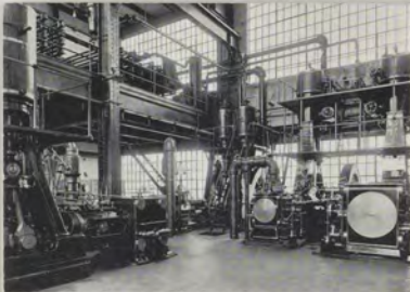
Part of the refrigeration department
